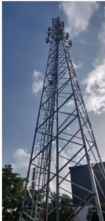
Bangalore - Roof Top Tower Tippenahalli
